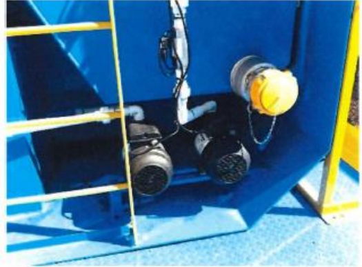
One of these NOV Mono pumps pressurize final waste through the filter and onto the UV filter before irrigating onto the ground while the other returns sludge back into the system to allow another process step
